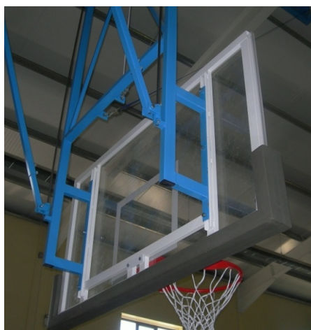
Fig. 2 Drop down goal support structure example
